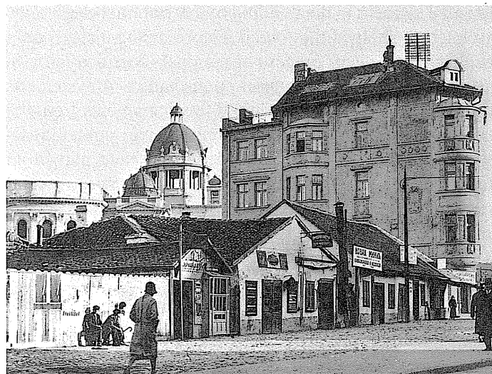
Fig. 2. The view from Dečanska Street in Belgrade, end of the 1920's (picture postcard from 1930)
