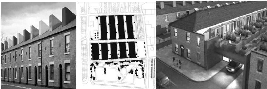
Image 1 | Front view of renewed row-houses (taken from: http://www.hdawards.org/ )
