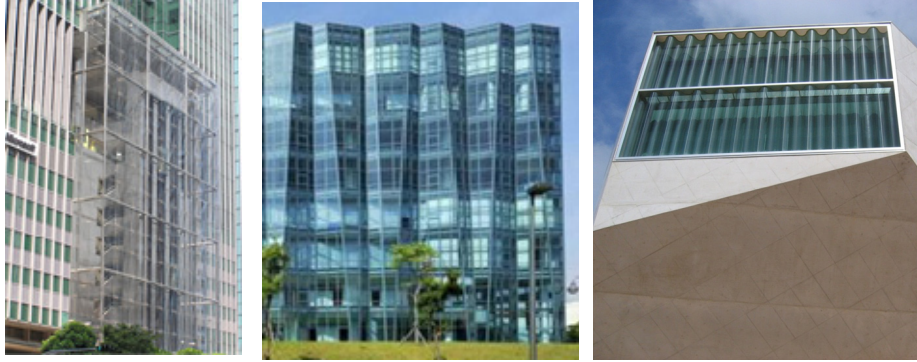
Figure 1a, b and c: Examples of different geometry of structural glass facade
