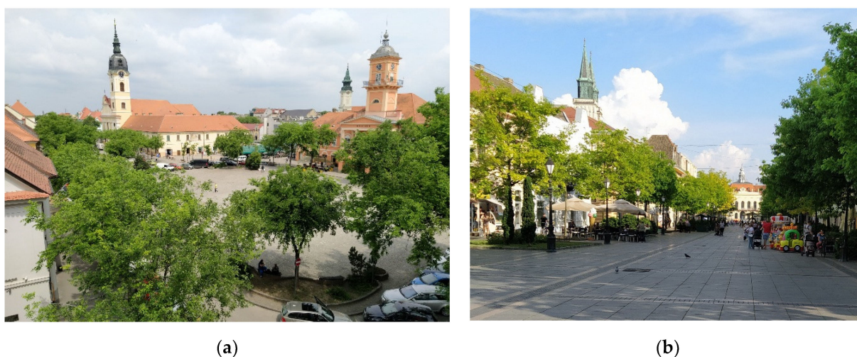
Figure 3. The historic core of Sombor: (a) The Square of Holy Trinity with the city hall and Roman Catholic Church; (b) the main pedestrian street and the backbone of the former Serbian Quarter with the “Županija” Building (District Court) in the background (author: B. AntoniĆ, 2023).
