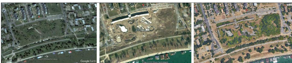
Figure 4 – Location of recreational complex in: 2001 (before construction), 2008 (under construction), 2022 (current state)
