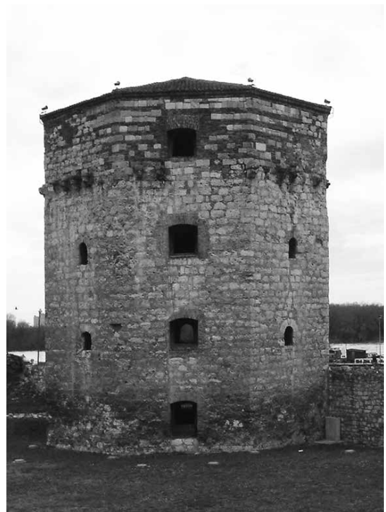
Figure 3. Nebojša Tower before the interventions https://commons.wikimedia.org/w/index.php?curid=730518
