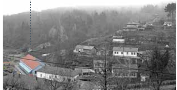
Figure 2. Senjski rudnik, under construction source Aleksandra Đorđević
