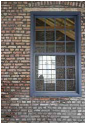
Figure 6. Mechanical workshop / Workshop space Source: Aleksandra Đorđević
