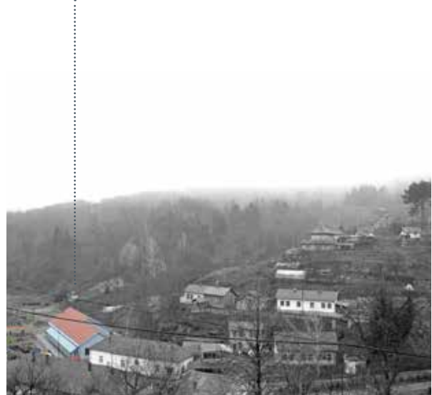
Figure 2. Senjski rudnik, under construction source Aleksandra Đorđević
