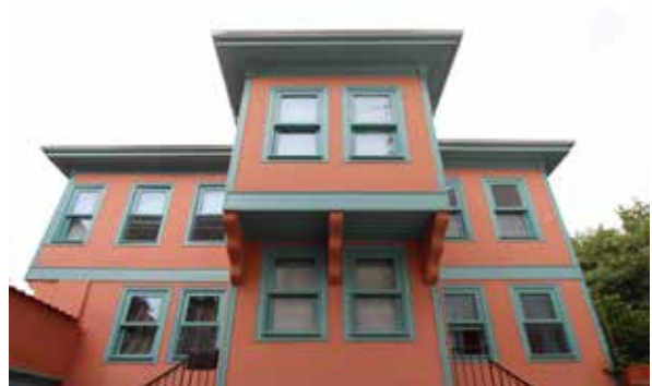
Figure 1. View of the historic building
