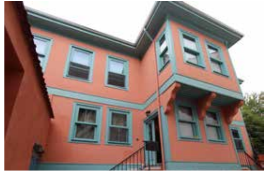
Figure 9. View of the main facade after the restoration.
