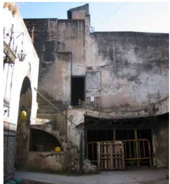
Figure 4. State prior to the intervention
