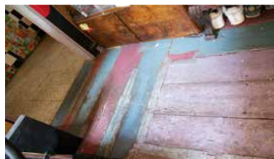
Figure 5. The building before the restoration (detail of the interior). Source:
