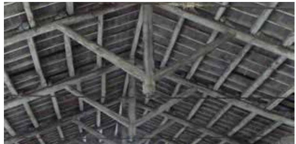
Figure 8. Attic trusses system before the intervention, 2011-2012.
