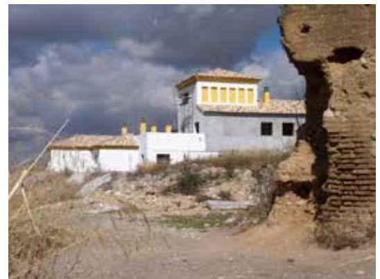
Figure 4. View of the breakage of the wall.
