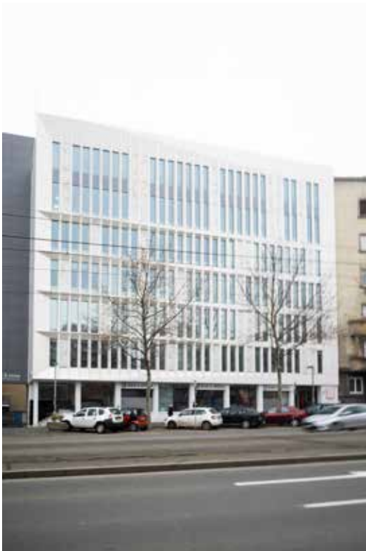
Figure 9. The office building after restoration source Aleksandra Dorđević
