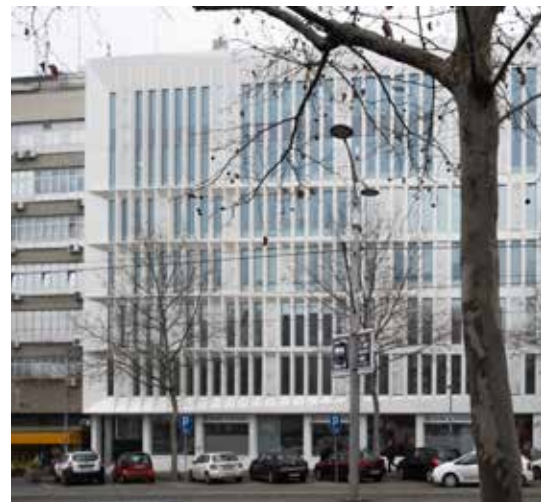
Figure 2: The office building
