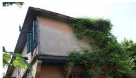
Figure 3. The building before the restoration (view from the street). Source:
