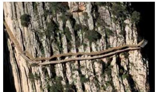
Figure 7. Aerial view of the two footbridges.
