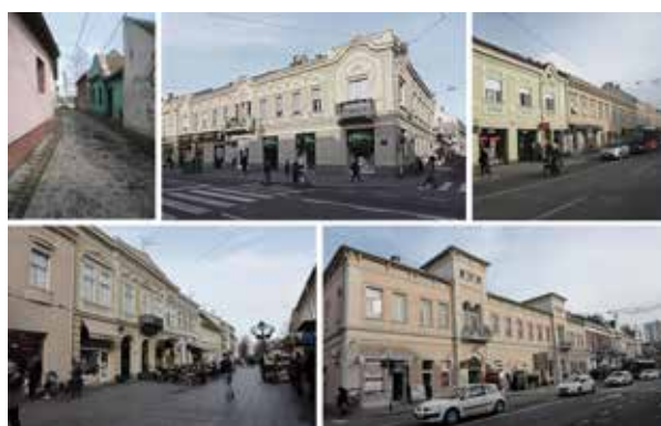
Figure 9. Urban Streets and facades after reconstruction source: authors of the case study
