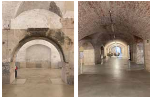
Figure 13 and 14. Former Bakery interior: ground floor. 2021.
