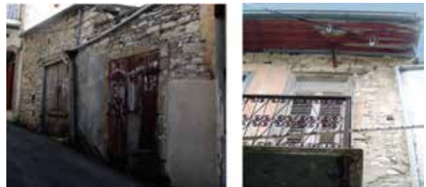
Figure 3. Situation before restoration works https://www.rehabimed.net/2015/11/urban-landscape-rehabilitation-in-lefkara-cyprus-the-recuperation-of-a-modern-past/
