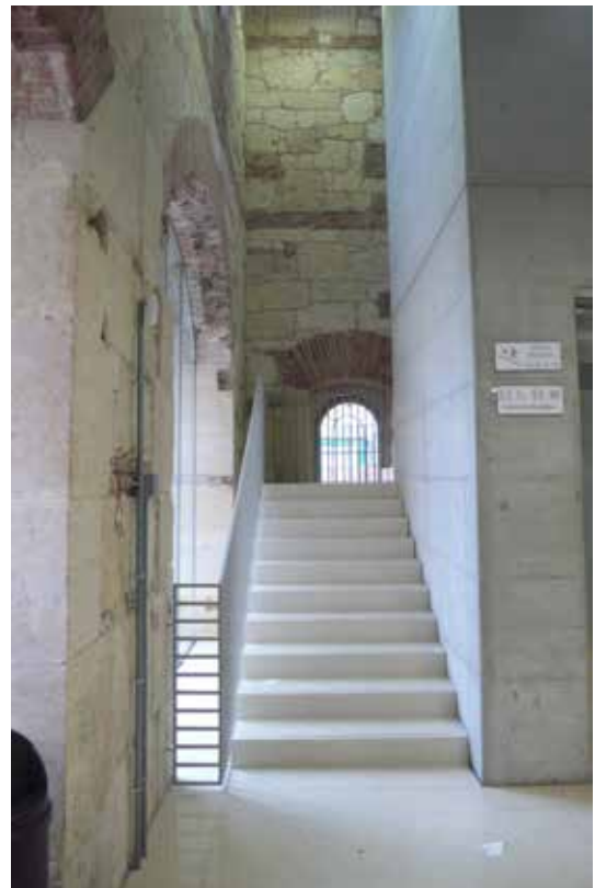
Figure 9 and 10. Interiors of Silos. Office boxes, study spaces and stair systems. 2012 Credit: Prof.ssa Emanuela Sorbo
