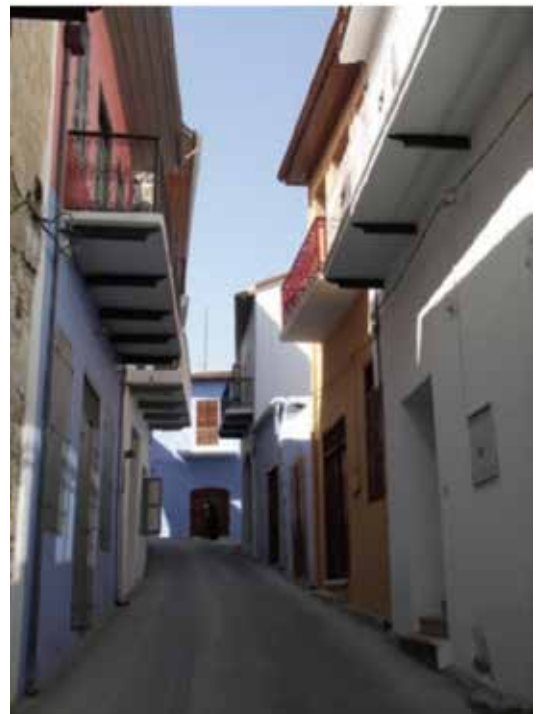
Figure 1. Situation after works
