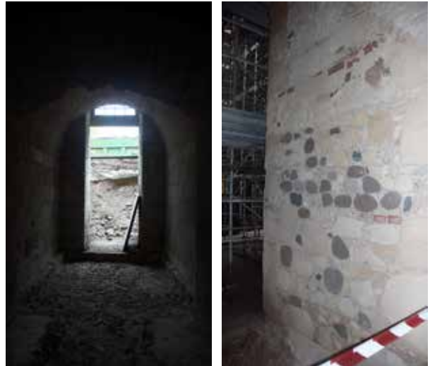
Figure 6 and 7. Basement, diamond blade enlargement of the opening, 2011-2012, before the intervention.
