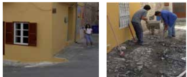
Figure 4. Situation before restoration works https://www.rehabimed.net/2015/11/urban-landscape-rehabilitation-in-lefkara-cyprus-the-recuperation-of-a-modern-past/
