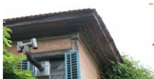
Figure 4. The building before the restoration (detail of the main facade). Source:
