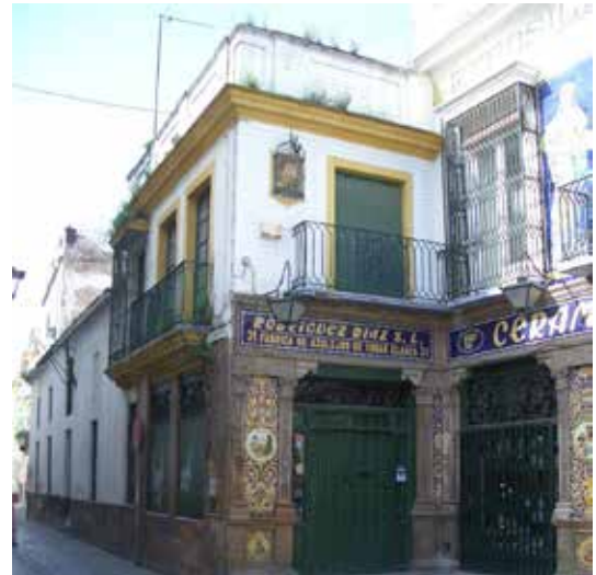
Figure 2. State prior to the intervention
