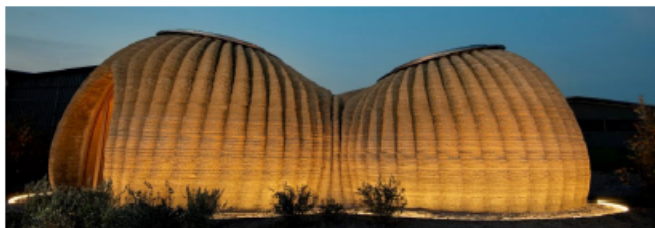
Figure 1 TECLA built prototype (source: https://static.dezeen.com/uploads/2021/04/tecla-3d-printed-home-mario-cucinella-architects_dezeen_2364_hero_7.jpg , accessed: 18.09.2023)
