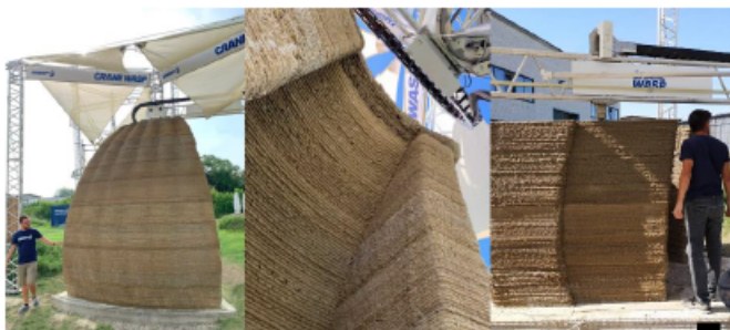
Figure 2 WASP technology printing process (source: https://www.3dwasp.com/en/3d-printed-house-tecla/ , accessed: 18.09.2023)
