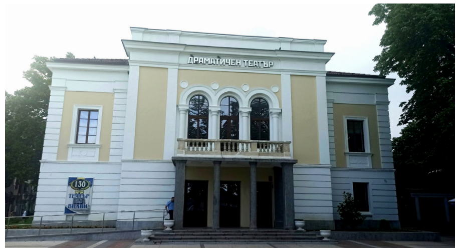
Fig. 027 / Middle-sized cities in Danubian states usually have some attributes of bigger cities, such as monumental buildings or important institutions. An example is a Drama Theatre in Vidin in North-western Bulgaria (Author: D. Mincheva-Yordanova, 2022)
