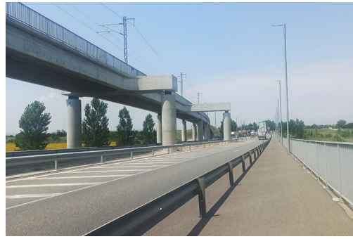
Fig. 255 / “New Europe” Bridge across the Danube bridge between Vidin, Bulgaria, and Calafat, Romania, combines road and railway (Author: Bulgarian Guide, 2022).
