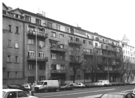
Figure 1: Building in Cvijiceva 112-120: street (North) façade – existing state
