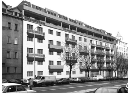
Figure 5: North façade – the first phase of reconstruction
