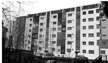
Figure 6: South façade – first phase of reconstruction
