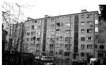
Figure 2: Building in Cvijiceva 112-120: court (South) façade - existing state
