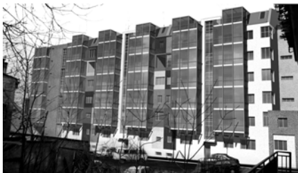
Figure 8: Reconstructed court façade – phase 2.
