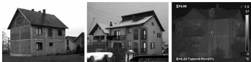
Figure 8. House type 2 and the thermo-vision photo of the construction (photo Ksenija Bunjak)
