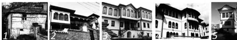
Figure 2. The spatial development of the Macedonian town house: 1) Štip, one-storey house; 2) Veles, two-storey house; 3) Wide Kruševo house; 4) Wide and simetrical Debar house; 5) Tall Ohrid house. (source: Authors)
