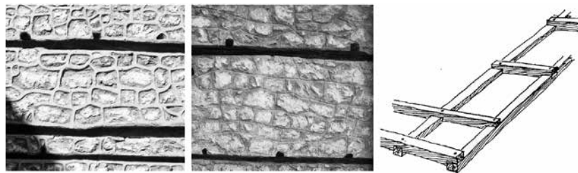
Figure 7. Type of finishings and stiffening of stone walls: a) Concaved mortar joints and visible cerclages; b) Convex mortar joints and visible cerclage; c) A system of wooden cerclages ( santrač ). (source: Чипан, Б. Старата градска архитектура во Охрид. Скопје: Македонска книга, 1982.)
