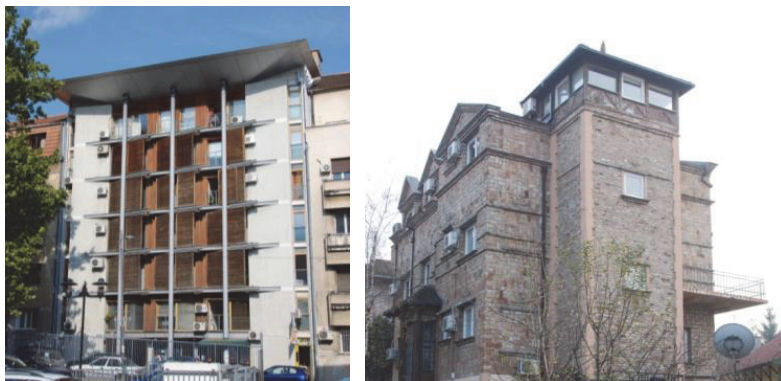
Figure 1. Wood as an element of façade cladding combined with other material (brick, artificial stone): a. Residential building on Milovana Marinkovica Street, b. Residential-business building on Kumanovska street.
