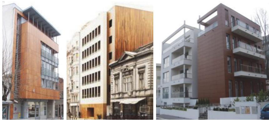
Figure 3. Composite material as a façade cladding: a. A building on Jagiceva Street, b. Residential building on Velisava Vulovica Street, c. "Square Nine" hotel at Students' square.
