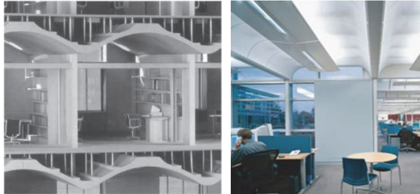
Figures 2 and 3. Arched reinforced concrete floor structure in Portcullis House, London, UK, 2001, designed by Michael Hopkins and Partners and in Wessex Water Operations Centre, Bath, UK, 2000, designed by Bennetts Associates. [Sources: Smith, P. F. (2005). Architecture In A Climate Of Change: A Guide to Sustainable Design . Elsevier/Architectural Press. 137; http://www.bennettsassociates.com/practice/sustainability/ ]
