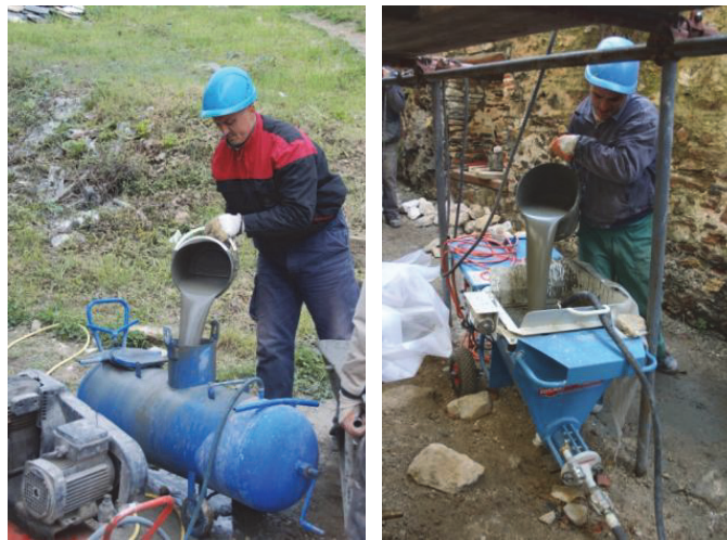
Figure 2. Injection equipment: a. Equipment with a standard closed drum, c. Injection machine with a spiral rotor
