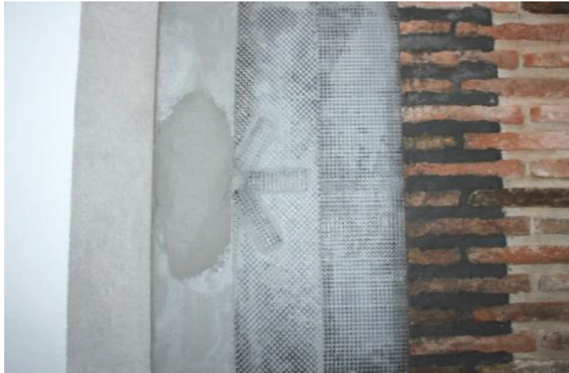
Figure 4. The phases of strengthening of walls using carbon meshes
