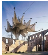
Figure 3: Primary steel structure of the protective membrane structure in the courtyard of the castle Kufstein.
