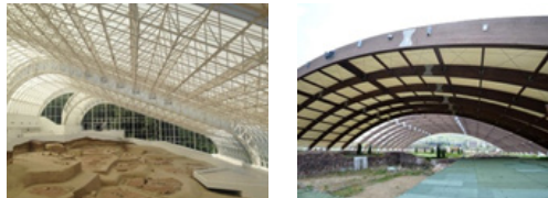
Figure 1: Permanent protective steel structure over the site in Lepenski Vir.
