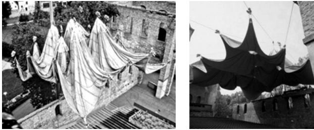
Figure 10: Opening / closing the textile membrane structure above the church yard in Bad Hersfeld.
