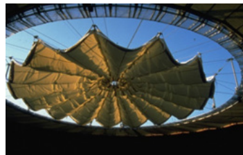
Figure 12: The membrane roof structure of the Bullring Arena (Zaragoza, Spain)
