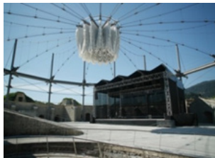
Figure 3: Primary steel structure of the protective membrane structure in the courtyard of the castle Kufstein.
