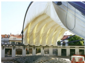
Figure 6: Fixed protective membrane structure, arena Nimes, France.
