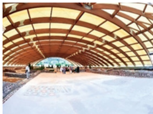
Figure 3: Primary steel structure of the protective membrane structure in the courtyard of the castle Kufstein.
