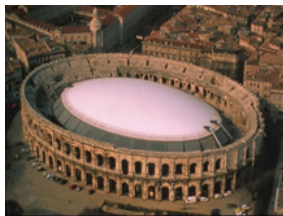
Figure 6: Fixed protective membrane structure, arena Nimes, France.
