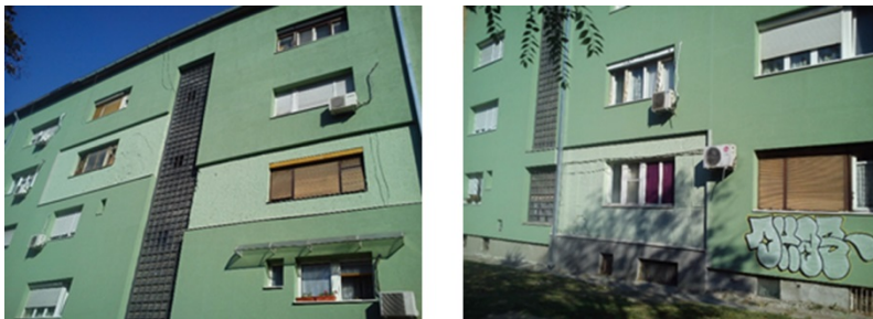
Fig. 1. Effects of partial thermal insulation of façade walls – example of a multifamily building from Belgrade
