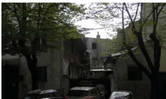
FIGURE 3 Typical examples of low-income and upscale inter-war housing in central Belgrade, with the problem of poor maintenance in both cases today
