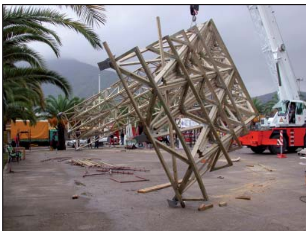
Figure 10. Lifting the prototype of construction with a car crane
