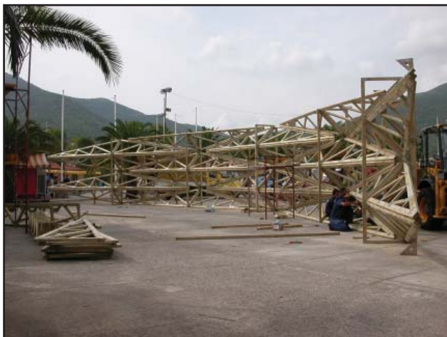
Figure 9. Installation of cylindrical folded construction on the ground
