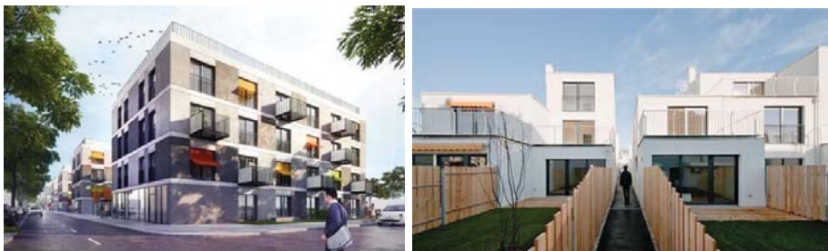
Figure 19 and 20. Middle-density housing projects in Aspern, Austria (source: Kirsch ZT; Detail Press)
