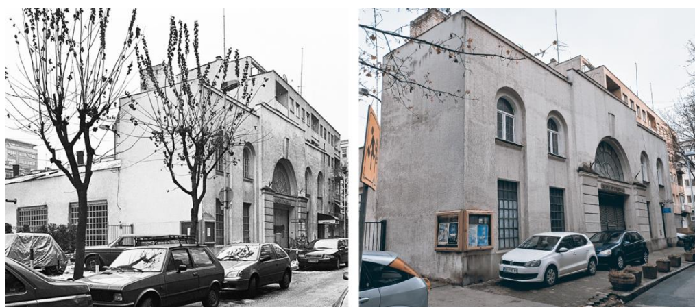
Figure 17. The First Modern Garage in Belgrade ( Left —previous state, source: The Cultural Heritage Protection Institute of the City of Belgrade, link: https://beogradskonasledje.rs/wp-content/uploads/2022/09/00-glavna-146-1024x639.jpg , accessed on 15 January 2024) ( Right —current state, provided by authors: Nikolić M., Ščekić J., Drobnjak B. and Takač E.).
