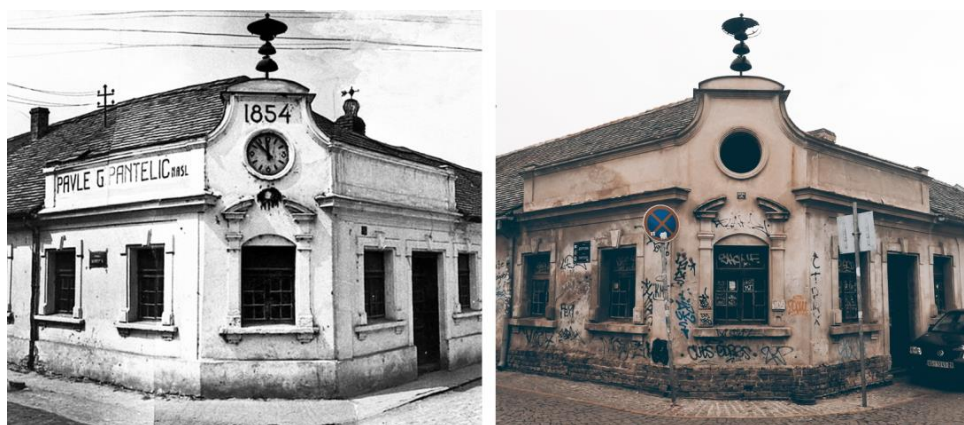
Figure 11. The Locksmiths’ Workshop and Foundry Pantelić (Left—previous state, source: The Cultural Heritage Protection Institute of the City of Belgrade, link: https://beogradskonasledje.rs/wp-content/uploads/2022/08/00-glavna-61-1024x604.jpg , (accessed on 15 January 2024)) (Right—current state, provided by authors: Nikolić M., Šćekić J., Drobnjak B. and Takač E.).
