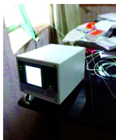
Figure 6. The set-up of sensors for internal wall surface temperature, wall No. 1
