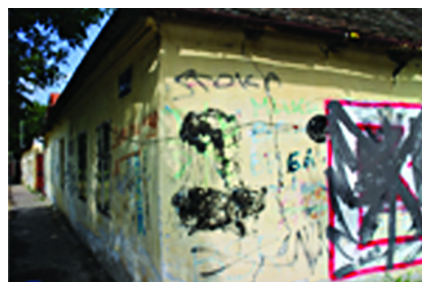
Figure 7. The set-up of sensors for outdoor wall surface temperature, wall No. 1
