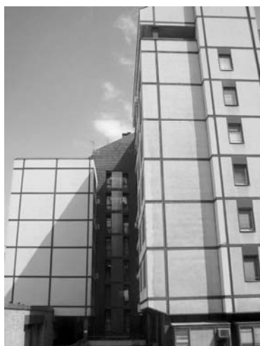
Fig. 9. The Lateral Façade -the photograph
