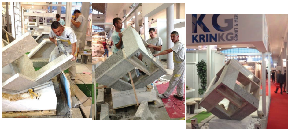
Figure, 8: Construction of the Box Packing structure of natural stone and the final installation at the Belgrade Stone Expo 2016
