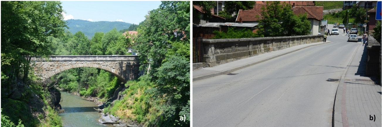
Figure 2. Masonry stone arch bridge in Ivanjica in its natural surroundings (a) and the traffic road of the bridge (b).
