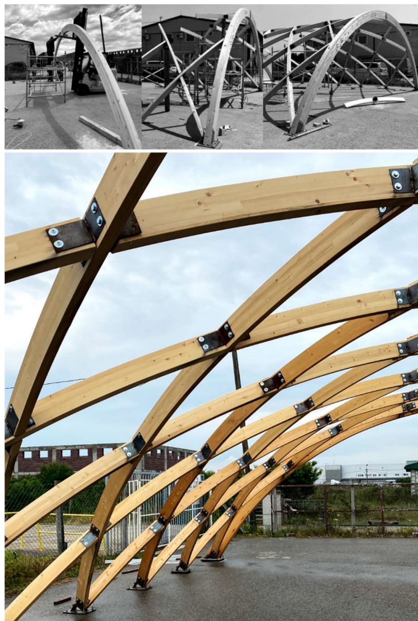
Figure 14. Photo of the construction process and the physical model in detail.
