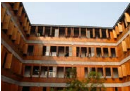
Figure 5. Cedar wood boards for courtyard façade (Building No. 5)
