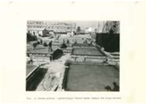
FIG. 5: The production of floor slabs for the IMS system at an Experimental housing construction site, album of the Department of Concrete (II) 1960, IMS Archive.
