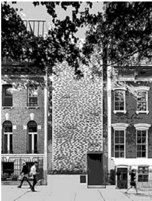
Fig. 10 Residential building East 51st Street, New York, USA, designed by Peter Gluck and Partners, 2009. Author's elaboration on the basis of illustration published in: http://www.bryla.pl/bryla/56,85298,10474730,Miejskie_plomby.html
