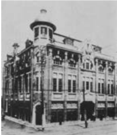
Figure 1 Maruzen Book Store, Nihombashi, Tokyo, completed in 1909.
