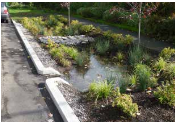
Figure 2. Green street planter after a rain in Portland, Oregon,
