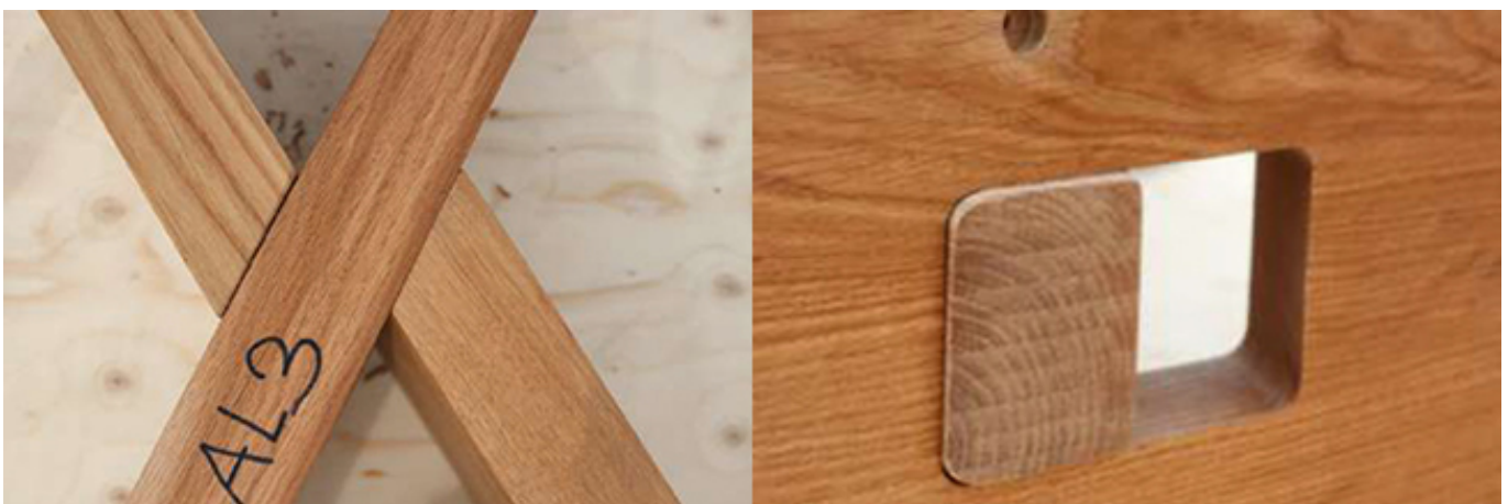
Figure 8. The wood joint for a classical pitched roof with a lamella diamond pattern. The left photo shows the joint in plan, and the right shows the elevation with one connecting lamella in place [27].
