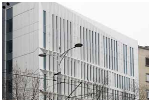
Figure 8. The building facade - after the restoration source Aleksandra Đorđević
