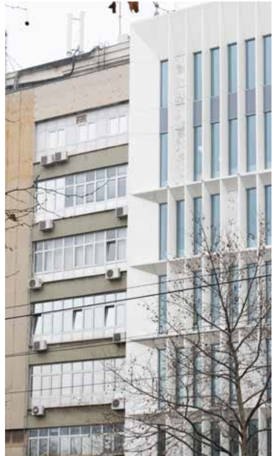
Figure 7. The building facade - after the restoration source Aleksandra Đorđević
