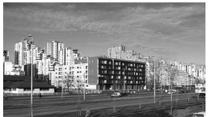
Figure 3. Group I-B, Social non-profit housing in PFC 10, Jurija Gagarina Street, Block 61, New Belgrade
