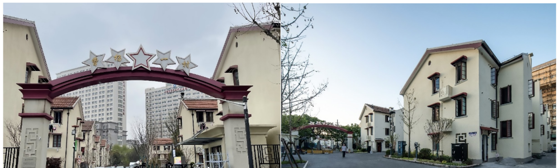
Figure 9. Caoyang No.1 Estate after renovation
