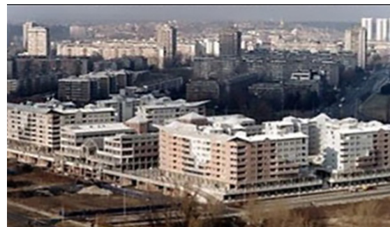
4Fs_FORTRESS_segregation ( http://ilicd.tripod.com ) TYPE 4 'Delevelling on the concrete' example
