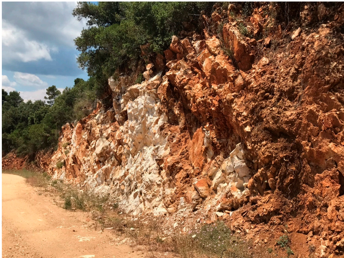
Figure 3. The stone deposit in a road-cut below Papa Konaki (provided photos taken by the author).
