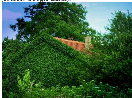
Figure 05. Building scale - House in green, Klek (source: Google Earth).
