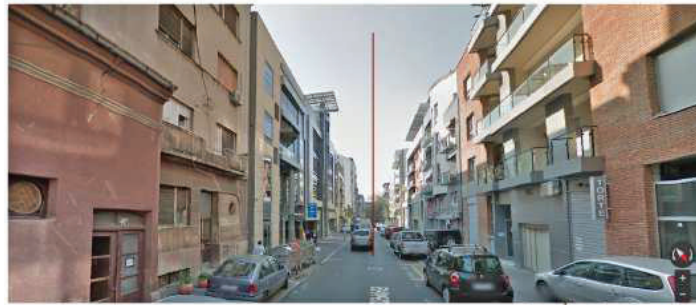
Fig. 8: The axis of symmetry on the street cross-section indicates the same height of the buildings across the street (Vasilev 2015)
