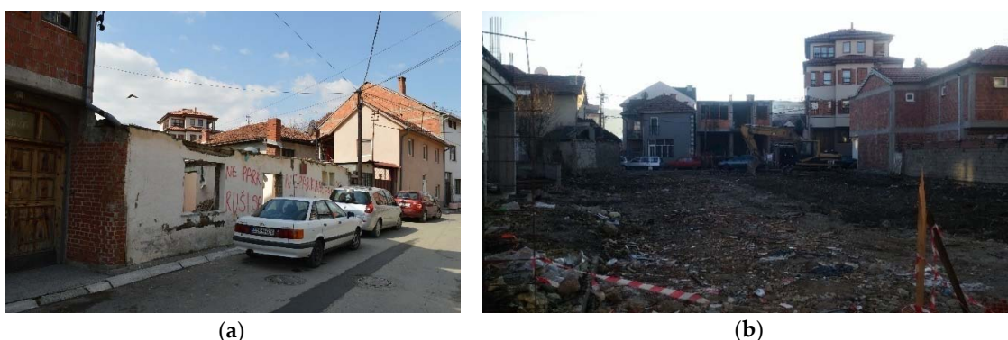
Figure 6. A cleared site for the construction of a multi-story building in the immediate vicinity of the historic center in the 7th of July Street (a) street view; (b) view of the lot.
