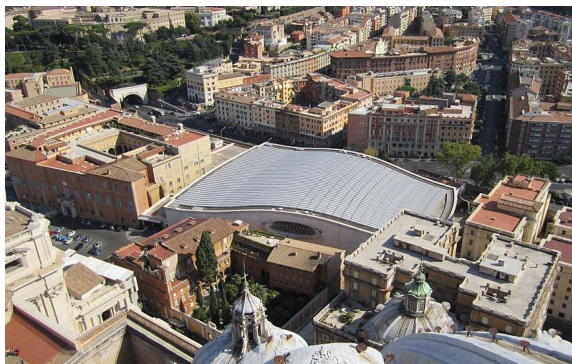
Figure 7: An example of PV application on an existing landmark object. Paul VI Audience Hall, The Vatican City (Pier Luigi Nervi, 1971) – awarded the 2008 European Solar Prize. https://en.wikipedia.org/wiki/Paul_VI_Audience_Hall
