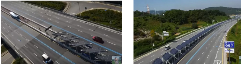
Figure 6: Bike line in the middle of a South Korean highway covered with solar panels. https://www.slashgear.com/bike-lane-in-the-middle-of-a-south-korean-highway-is-covered-with-solar-panels-16379387/
