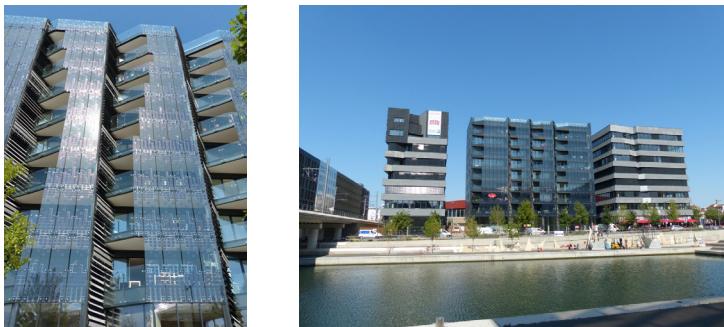
Figure 9: Example of an innovative approach to designing of PV facilities in a built environment. Kengo Kuma, Hikari Building, Lyon, France 2015, source of illustrations SADEV http://www.sadev.com/blog/vea-hikari-lyon-france/?lang=en
