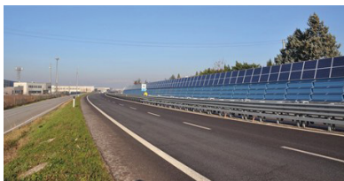
Figure 5: Sustainable design of road equipment. Sound barrier in Rome – left, http://www.worldhighways.com/sections/irf/features/photovoltaic-noise-barriers/ ; Solar-powered petrol pump – right, http://www.aurarays.com/solar-power-application .
