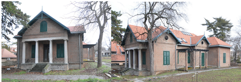
Figure 2: The residential building, Belgrade, the original appearance: North-west façade (left), South-west façade (right) (photos taken by the author)
