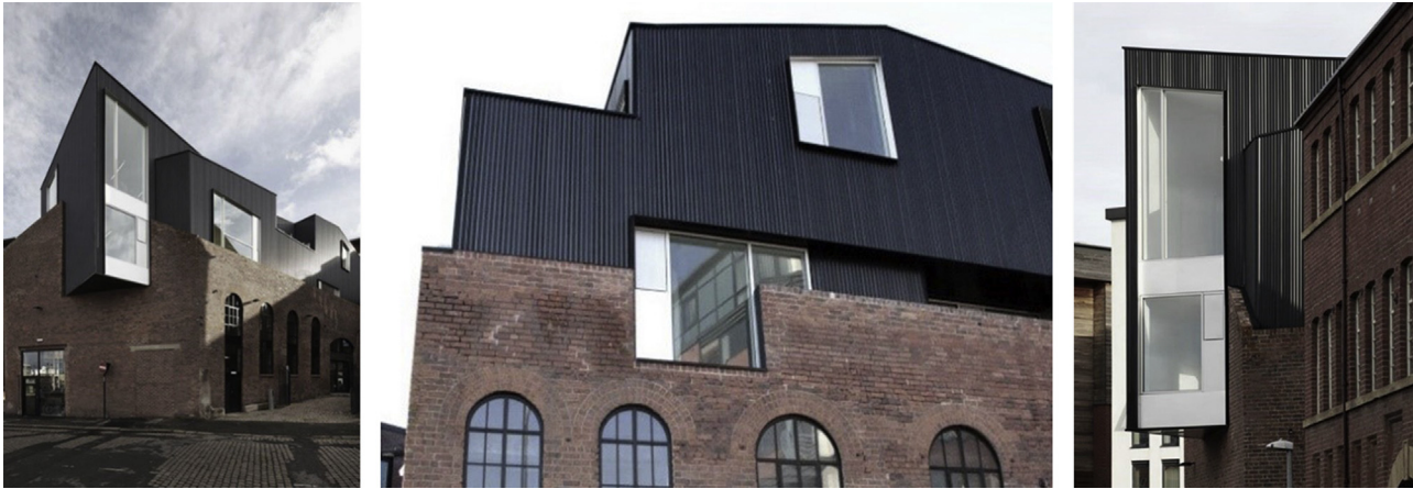
Figure 6 192 Shoreham Street, exterior of the building after the intervention. Source: Hobhouse (2012).
