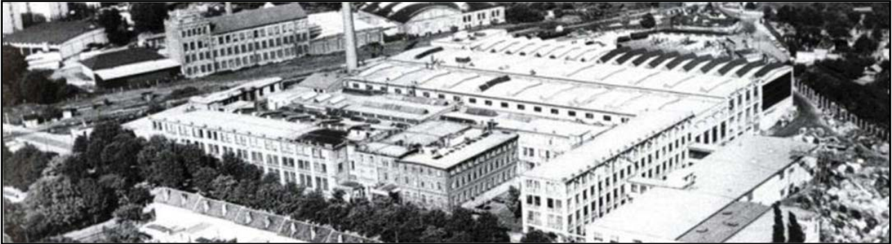
Figure 2: Ex-cable and wire factory in Vienna, Austria
