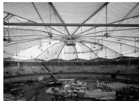
Figure 4 – Olympic arena under construction
