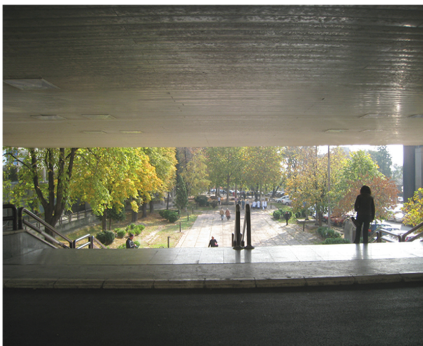
Figure 9: View of the pedestrian access to the central Polyclinic building, personal archive
