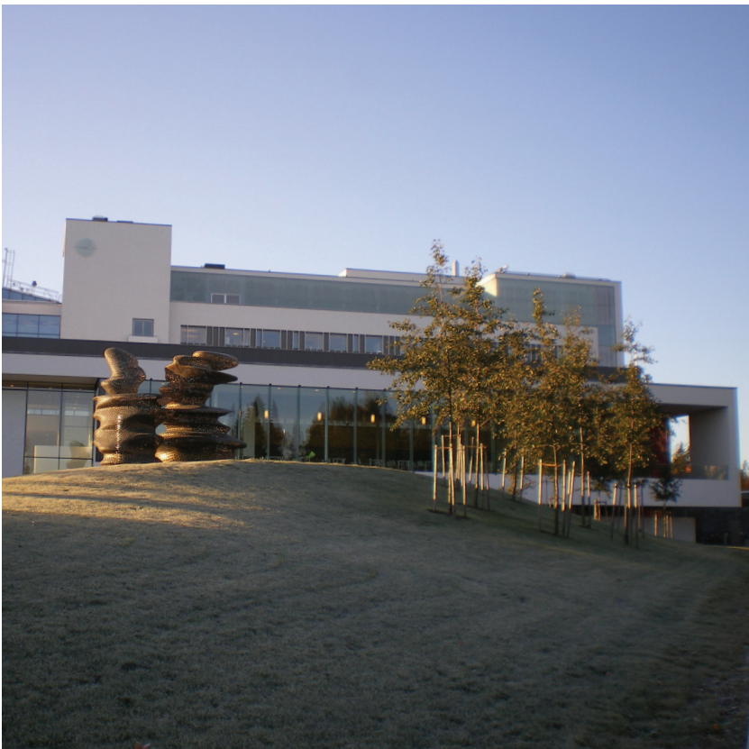
Figure 1: Outdoor spaces, Akershus University Hospital, Oslo, Norway, photo by Francesca Giofrè
