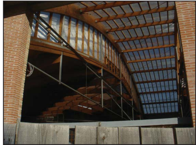
Figure 4. Sirmijum, Visitors center construction
