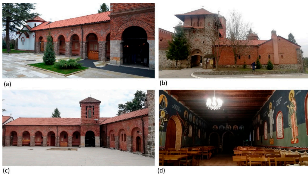
Figure 1. The Dining Room of the Žiča Monastery property: (a) appearance of the church of St. Sava and the Dining Room from monastery yard, (b) external appearance of the Dining Room and entrance of the monastery property, (c) appearance of the Dining Room from the monastery yard, (d) the interior of the Dining Room (provided photos taken by the author).
