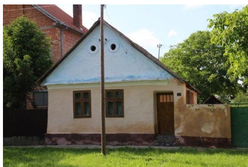
Figure 1. Traditional tree-part rammed earth house with porch
