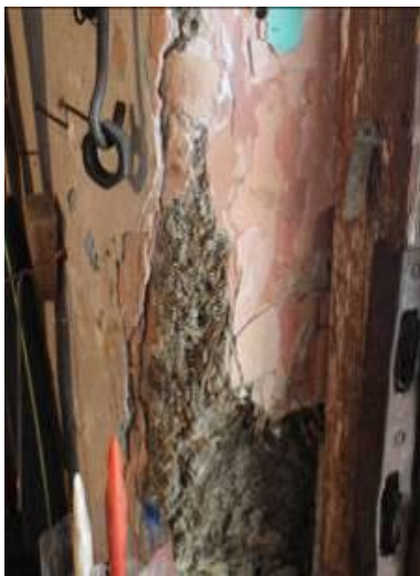
Figure 3. Rammed earth wall with a large quantity of added straw (chaff) plastered with mud mortar, a house in Vojlovica
