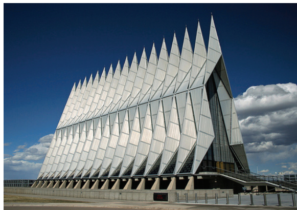
Fig. 4. Air Force Academy Chapel, Colorado Springs, USA, architect Walter Netsch, year 1962 [28]
