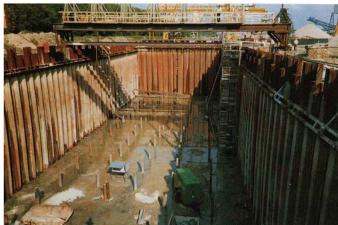
Fig. 7. Securing the foundation pit with Larsen planks [29]
