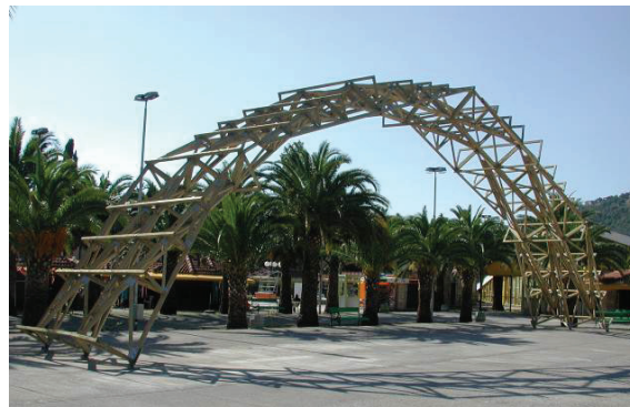
Fig. 11. Mounted prototype of cylindrical folded structure formed by using wooden trusses as the elements of folded structure, Fair in Budva, author architect Nenad Šekularac, Budva, Montenegro, 2005. [17]
