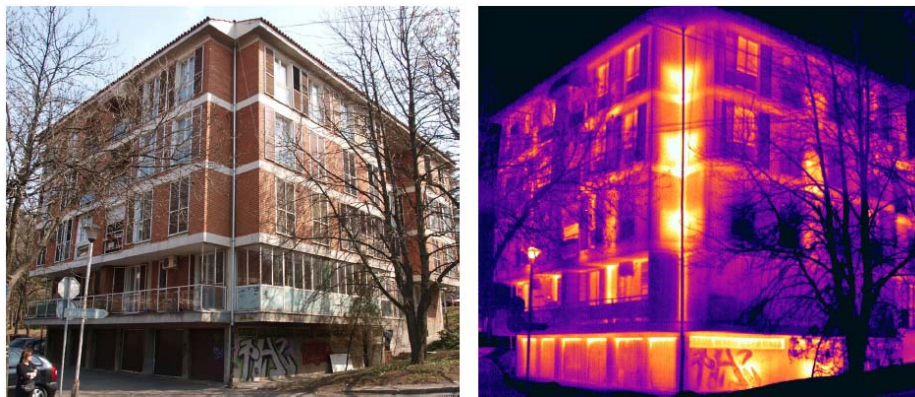
Figure 7. Housing in Košutnjak, Belgrade – conventional and IR image [5]
