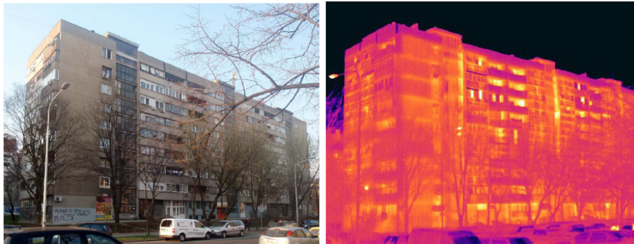
Figure 6. Block 8, New Belgrade – conventional and IR image [5]
