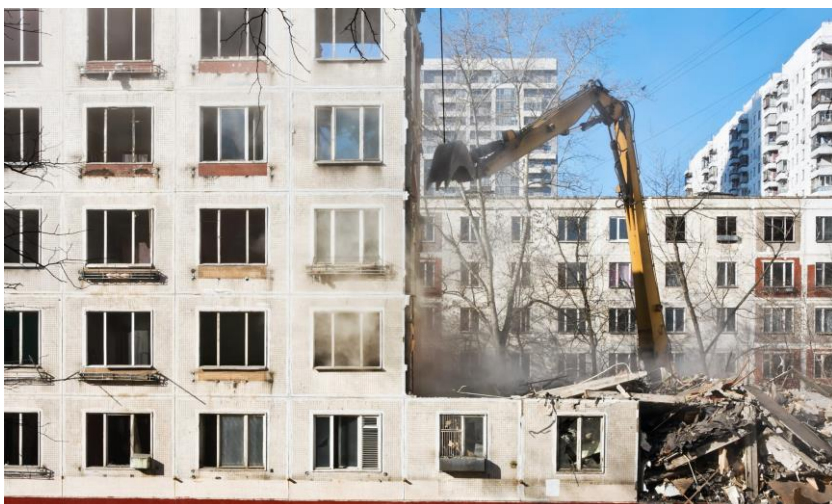
Figure 1: Khrushcheyvka standard types are classified into "disposable", with a planned 25-year life (сносимые серии) and "permanent" (несносимые серии). This distinction is important in Moscow and other affluent cities, where disposable Khrushcheyvkas are being demolished to make way for new, higher-density construction. Photograph: Andrei Makhonin/Tass
